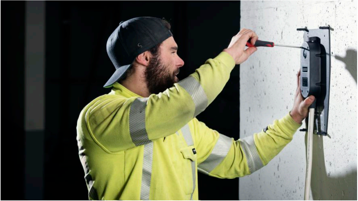
Installation of ZAPTEC charger backplate with certified partner
